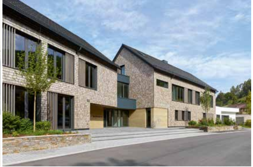
The restaurant of the Hotel Traube Tonbach by ARP Architekten is clad in wooden shingles.
