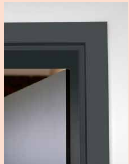
Detailed photo of the frame face.
