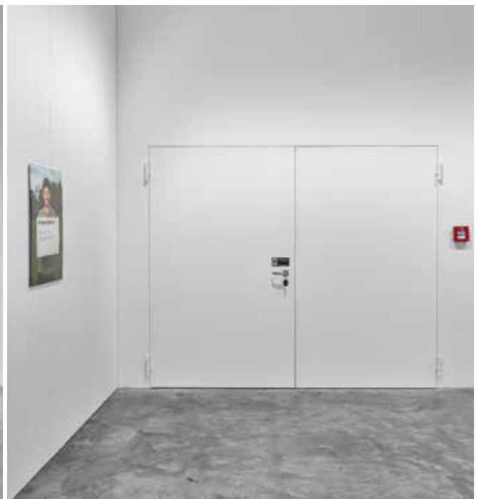
High-quality door view in detail: The double-leaf Hörmann steel construction project doors have a flush-fitting transition of the door leaves.
